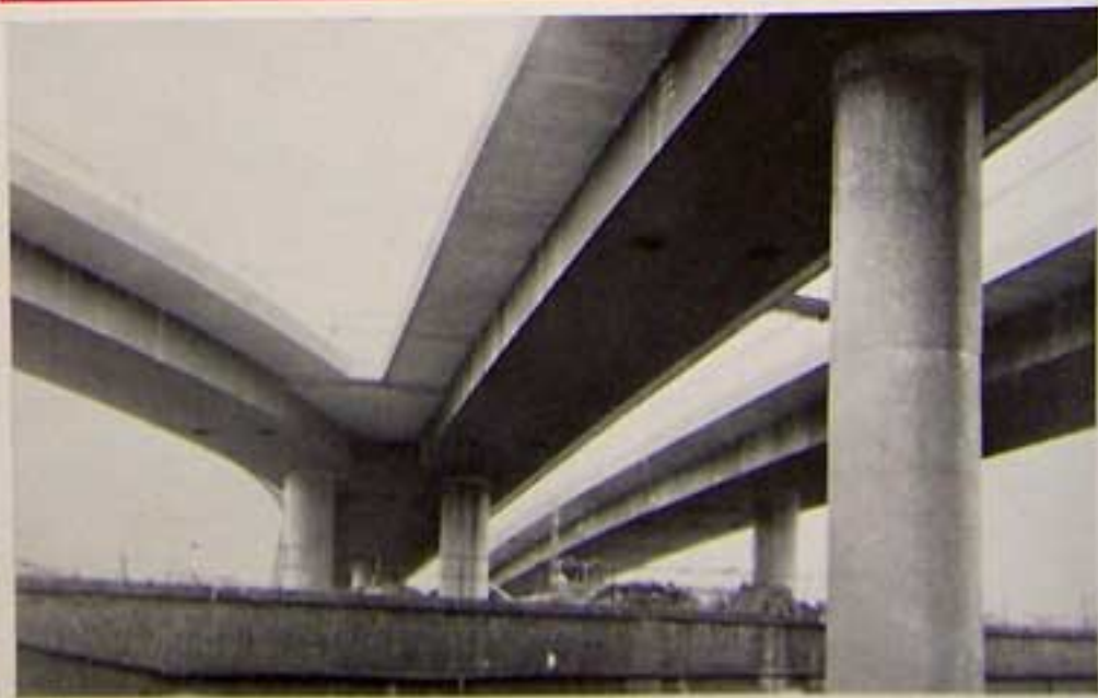
A photograph of part of the viaduct, during construction, which illustrates the relationship of the decks and columns.
