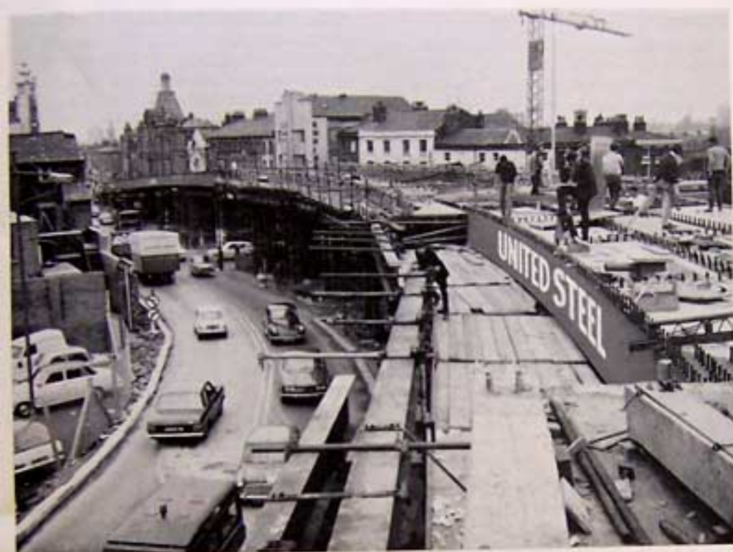
A view of one of the viaducts under construction showing the arrangement of trestles used to erect the steelwork.
