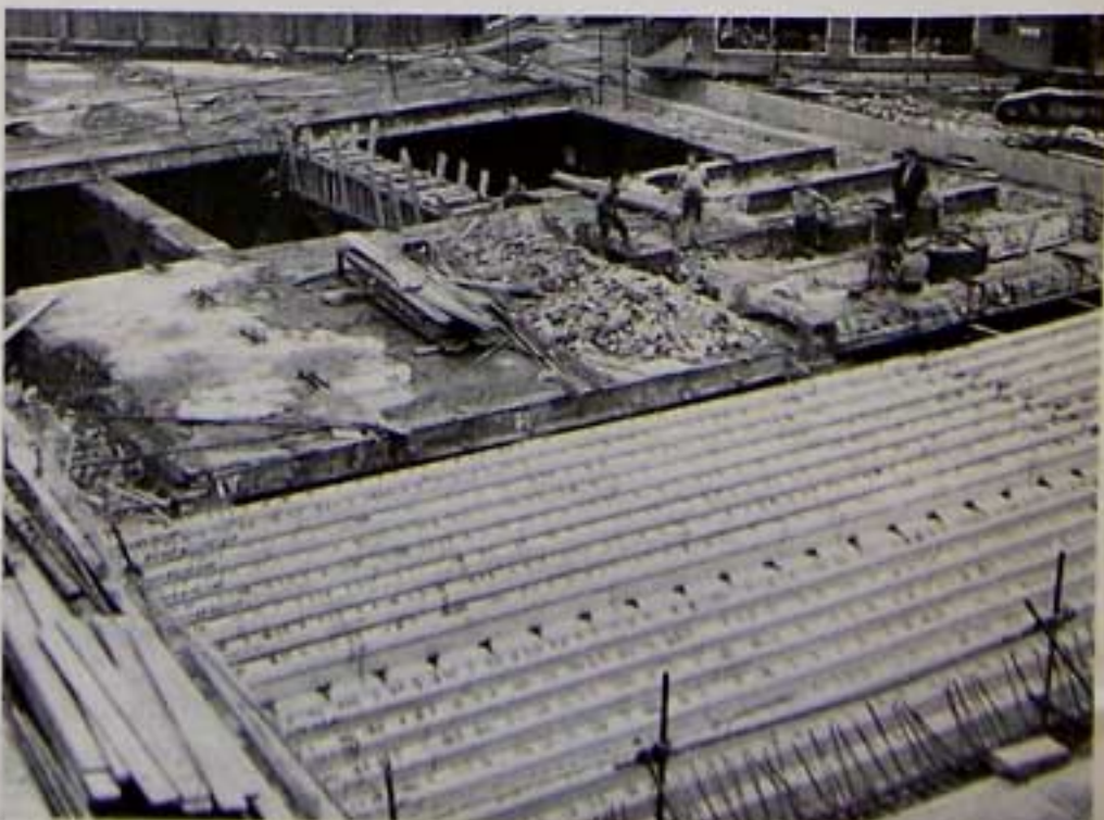
Progress picture showing the placing of the prestressed precast concrete beams during construction of the new roof to the Haymarket Railway Tunnel.
